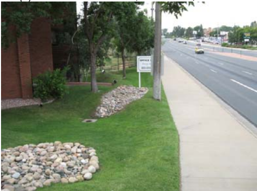
(3) Grade drainage retention/catch basin (west)
