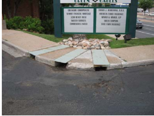
(2) Grade drainage @ parking lot
