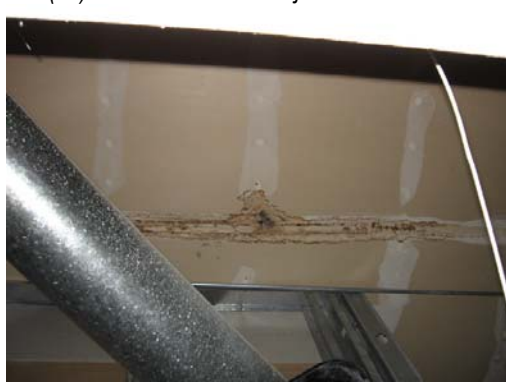
(22) Roof leak @ 7586 - 305
