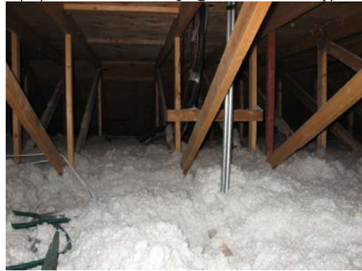
(14) Attic area w/loose fill fiberglass insulation
